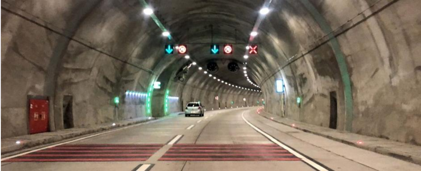
Çamlıca-Libadiye Tüneli, İstanbul
